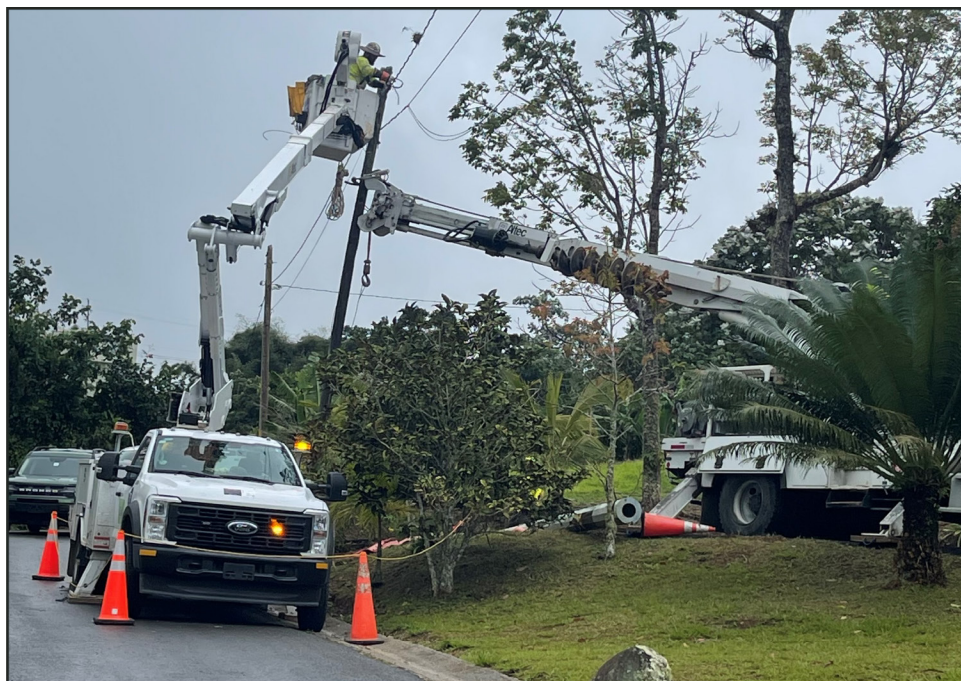
Figure 2: FEMA-funded Pole Replacement and Streetlight Repair Project in Coamo, Puerto Rico (February 2025)
