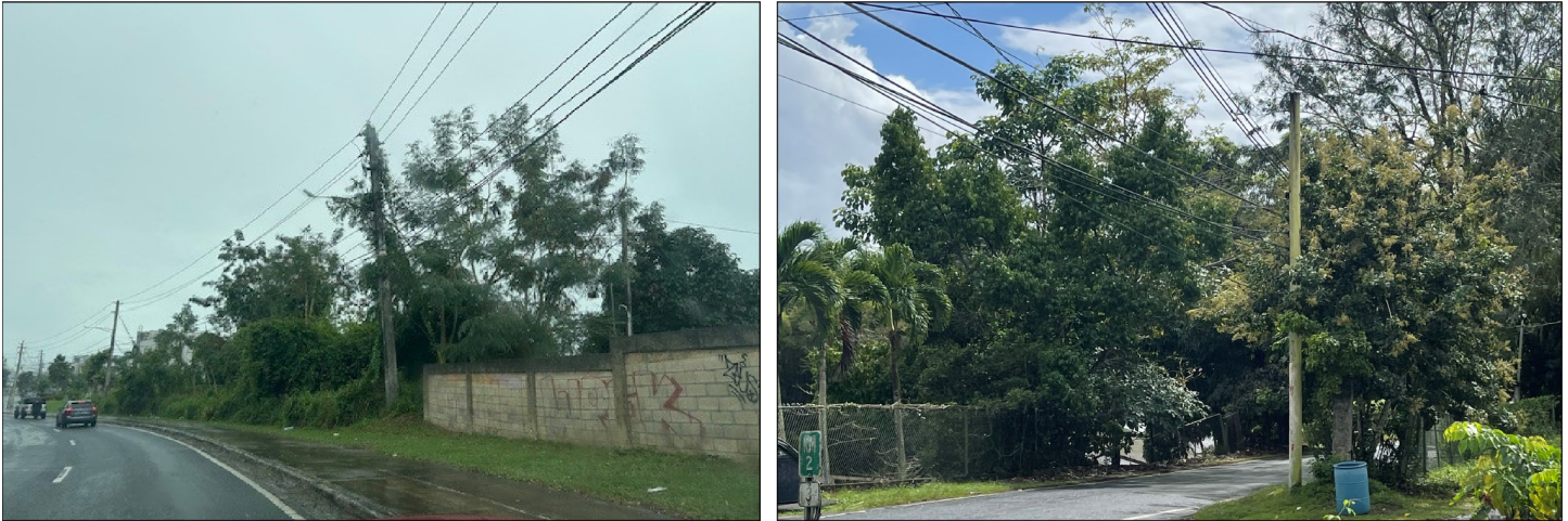
Figure 5: Examples of Overgrown Vegetation and Power Lines in Puerto Rico
