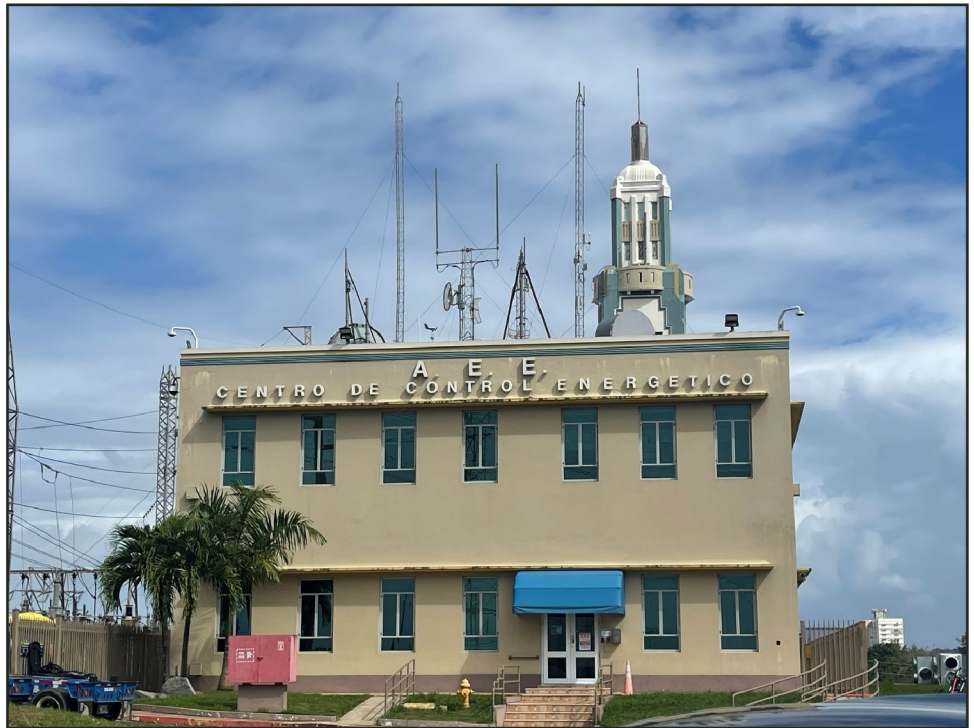
Figure 6: Monacillos Primary Control Center in San Juan, Puerto Rico (February 2025)
